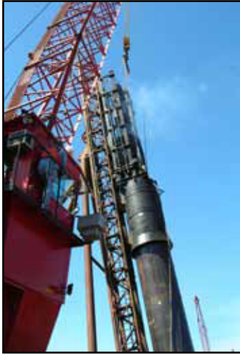
D225-42 With a 2.5 m Bottom Drive.
