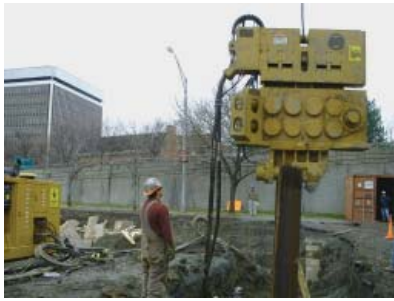
250VM with a sheet clamp driving sheets.
