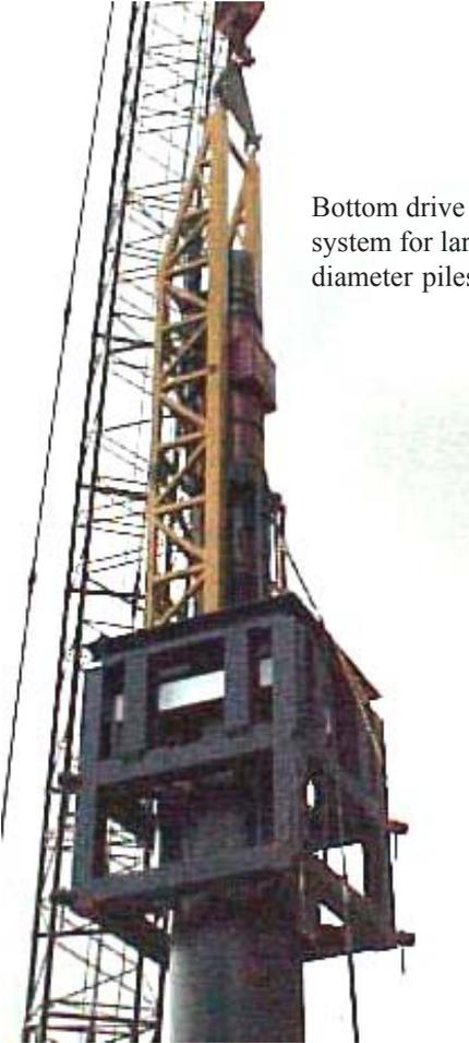
Bottom drive system for large diameter piles
