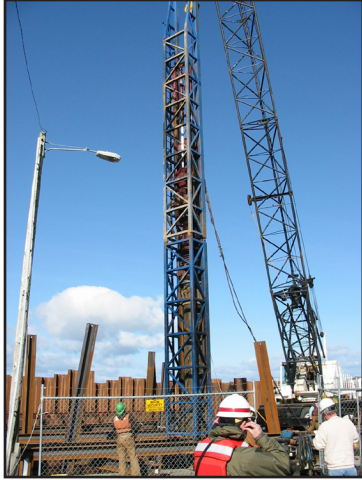
D36-26 Finishing Dolphin Piles.
