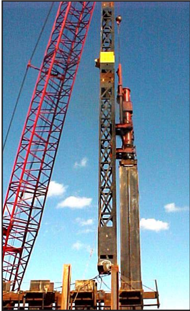
D62-42 in a stand-off driving Kingpile.
